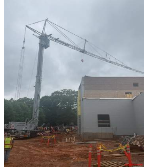
Crane lifting RTUs into place on rooftop
