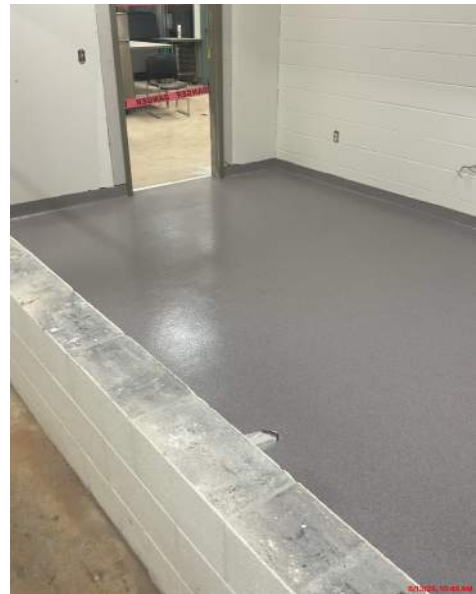
Epoxy Flooring Finished
