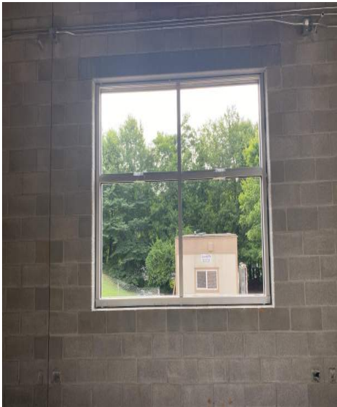
Window frame installed
